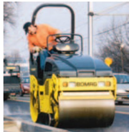
BW100AD-4 rolling a curbline.
